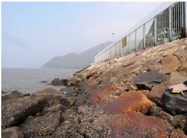
Coastal Area (Seawall)
