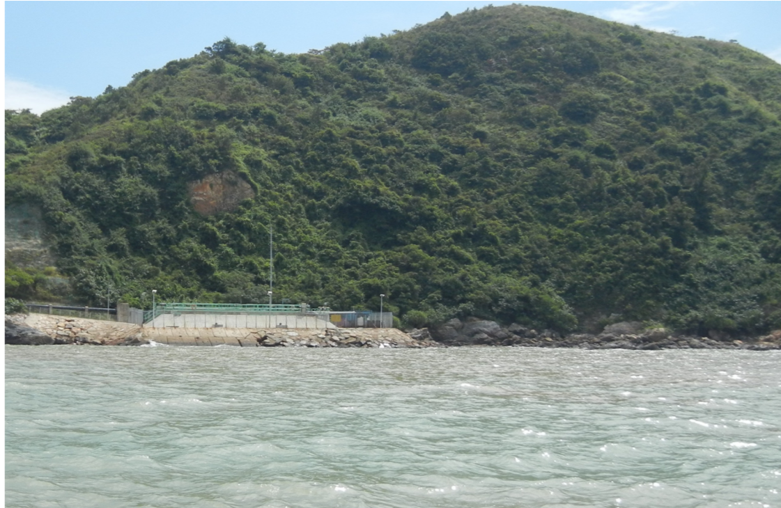
Existing View of the Existing Tai O STW
