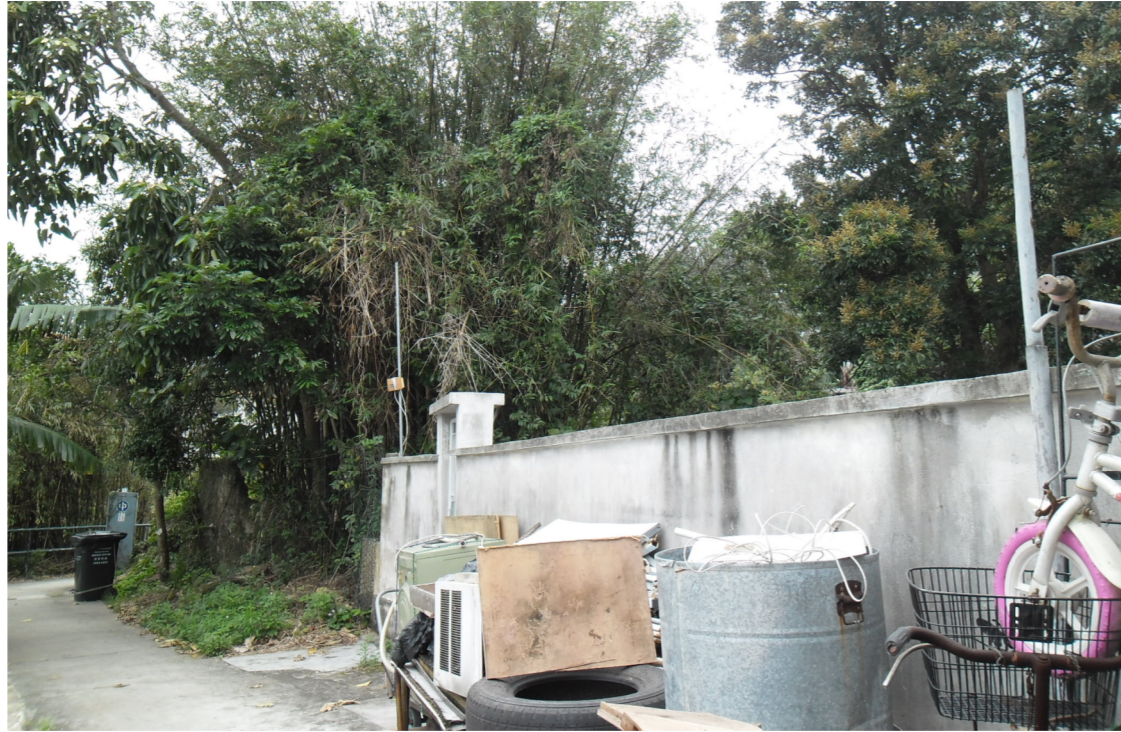
Existing View of the Proposed Fan Kwai Tong SPS Location
