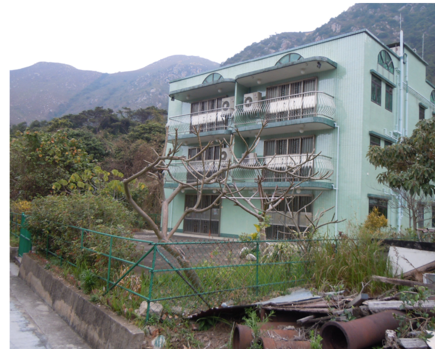
VSR HM-3 - Wang Hang Village
