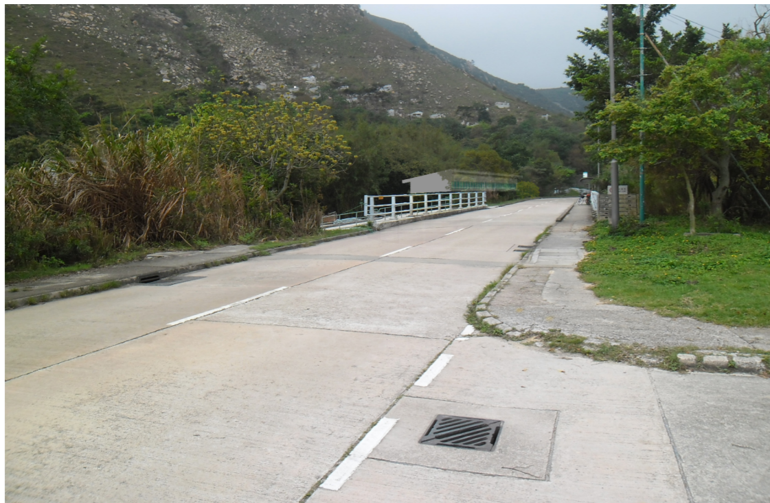
View of the Proposed Hang Mei SPS Upgrading - with visual mitigation measures - Day 1
