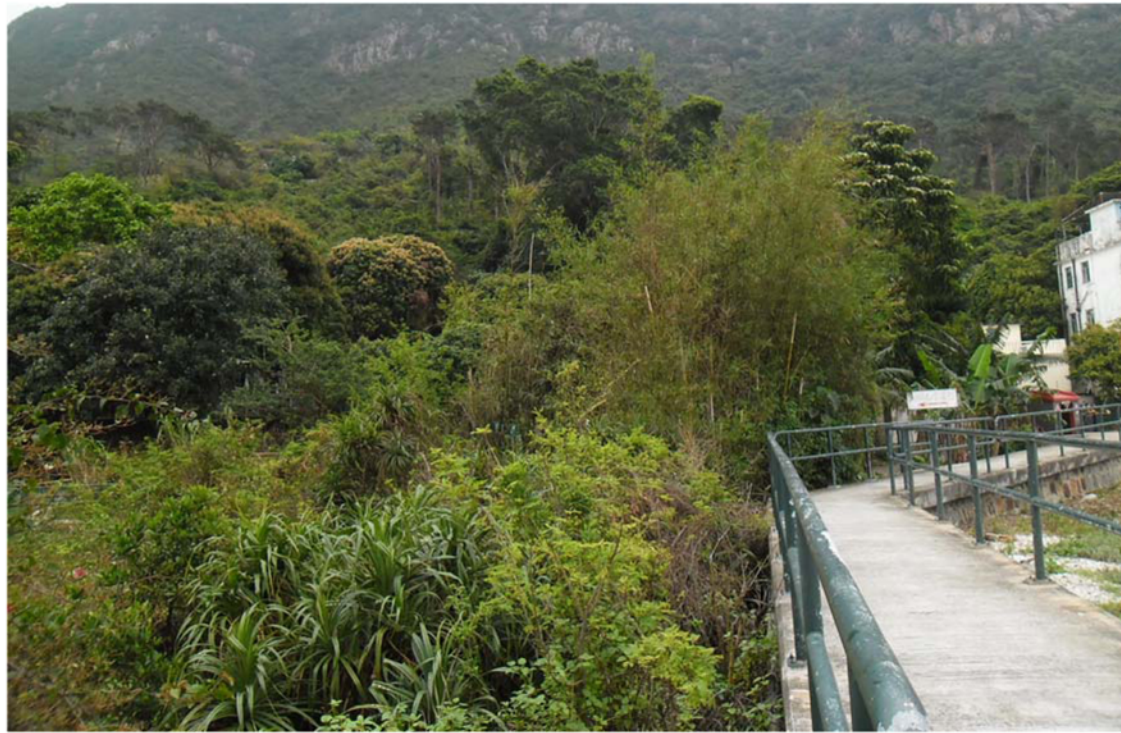
Existing View of the Proposed Fan Kwai Tong SPS Location
