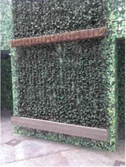
Hedera helix - temporary hoarding at Exchange Square
