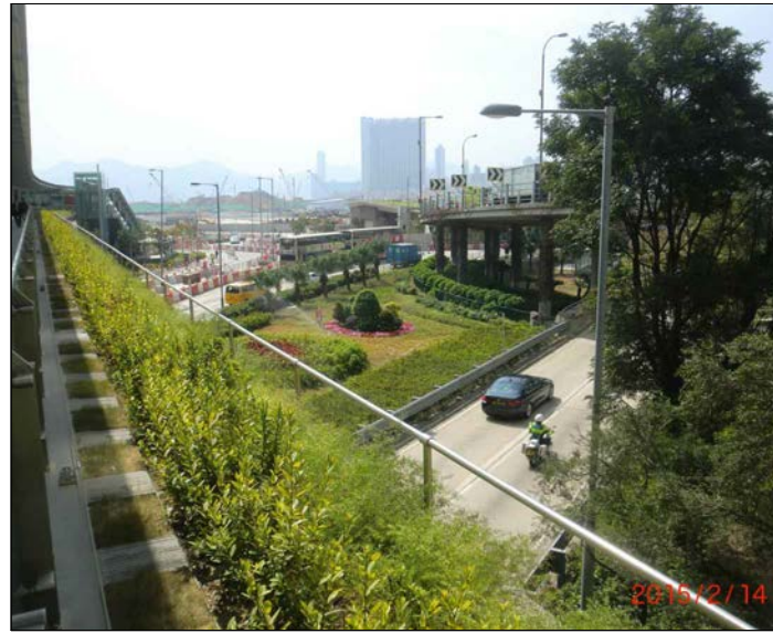
LR1-2: TREES IN AMENITY AREAS OF SAN PO KONG INTERCHANGE
