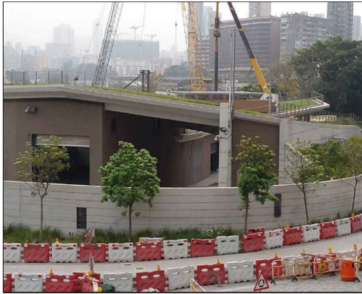
LR2-10: LANDSCAPE AT KOWLOON BAY PUMPING STATION #1
