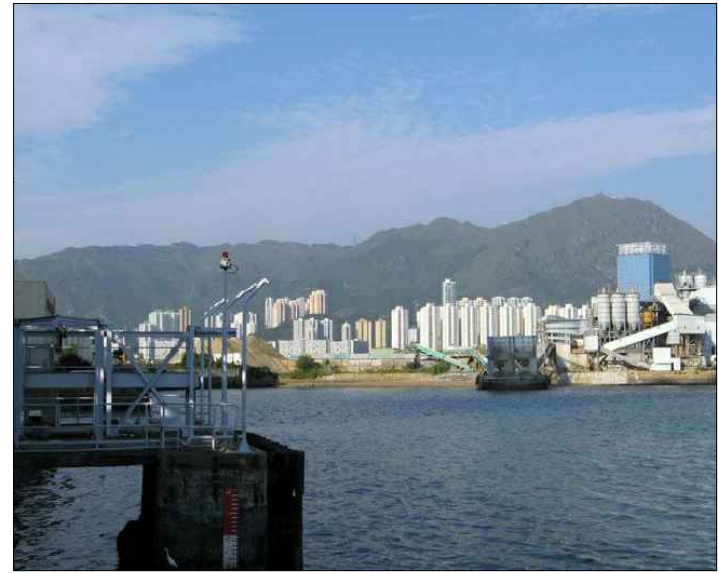
LR2-12: SEAWALL OF KOWLOON BAY TYPHOON SHELTER
