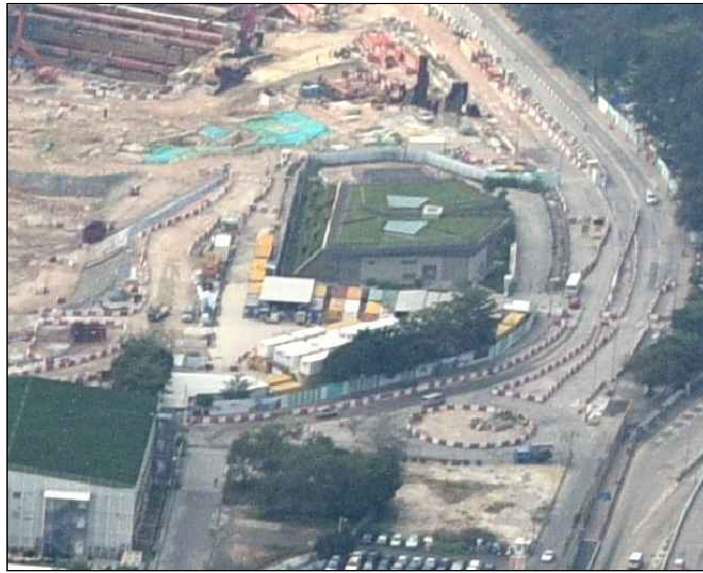
LR2-11: LANDSCAPE AT KOWLOON BAY PUMPING STATION #2
