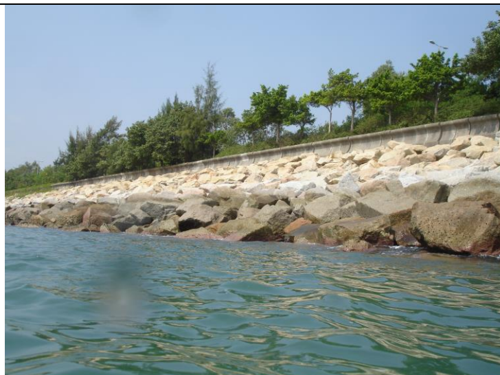
Plate 1. Station 1 at the artificial seawall at the Lamma Power Station.
