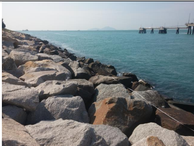
Plate 1 Lamma Power Station Extension artificial shore (Site A)
