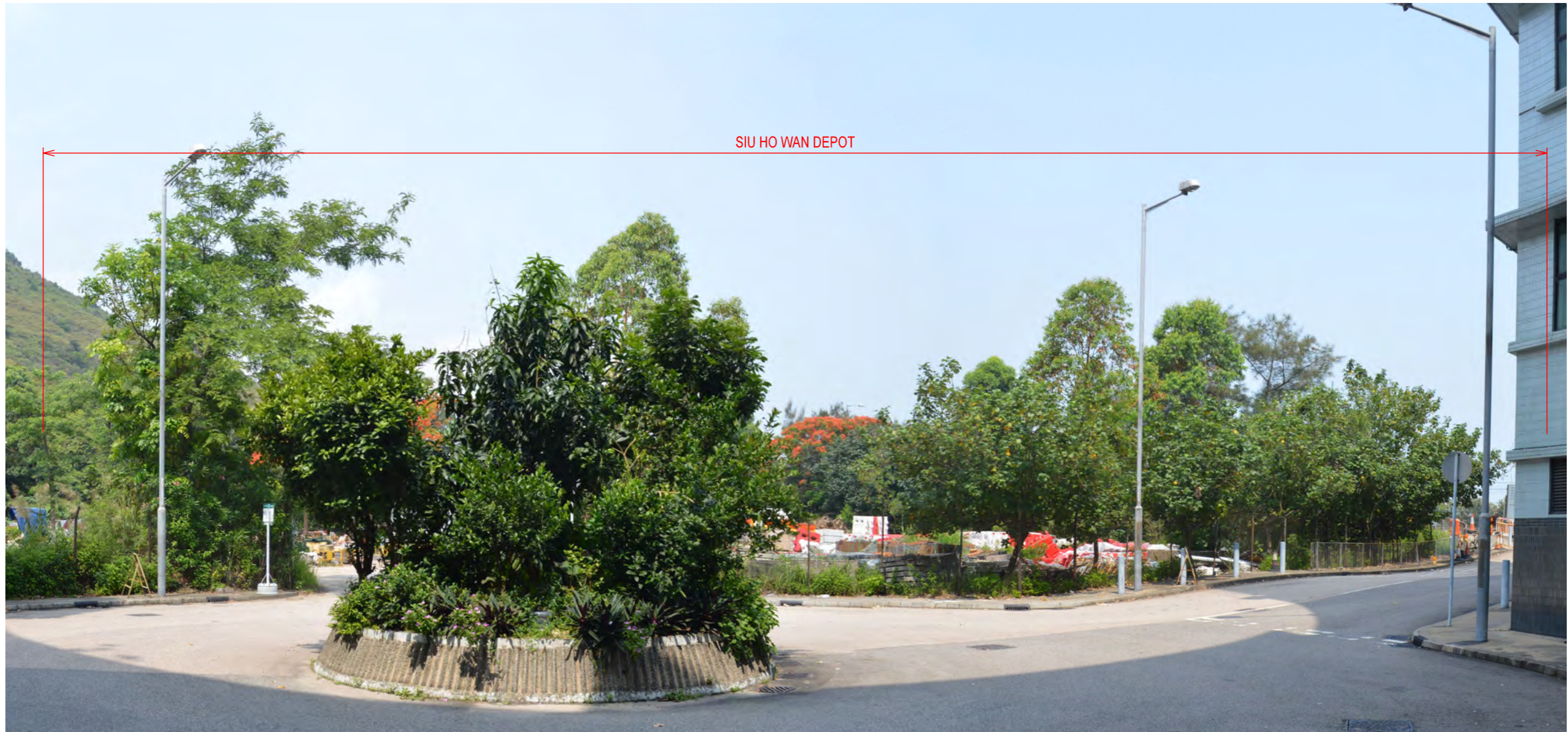
VSR 9 SIU HO WAN GOVERNMENT MAINTENANCE DEPOT (APPROX. 120M) TYPE OF VSR : OCCUPATIONAL
