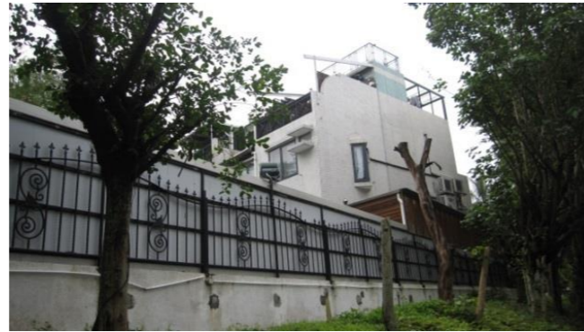
NSR 2 House No. 1, Narcissus Path, Palm Springs
