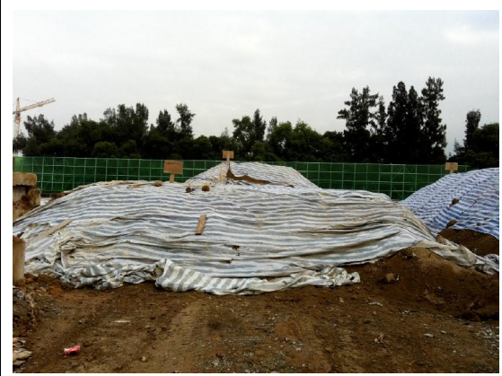
Photo 01 – The treated soil was covered with tarpaulin sheet and placed at a paved area for temporary storage.
