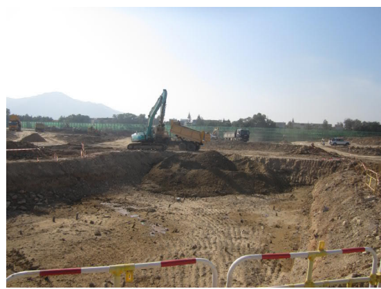
Photo 02 – The treated soil was started to backfill to the proposed location.
