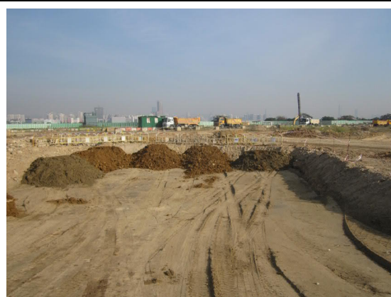
Photo 04 – The treated soil was covered by ordinary soil.
