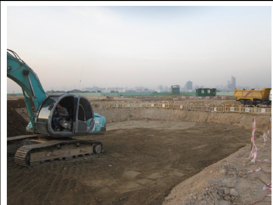
Photo 03 – All the treated soil was backfilled to the area.
