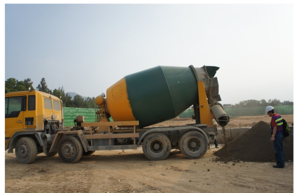
Photo 06 – Unloading of treated soil from lorry mixer.
