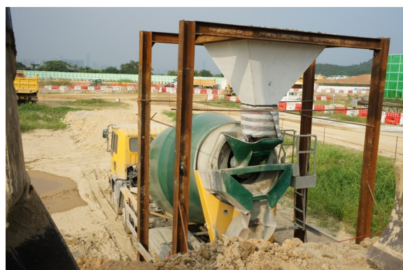
Photo 05 – Mixing in progress.
