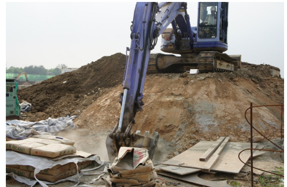
Photo 04 – Cement was added to the lorry mixer for the solidification process.
