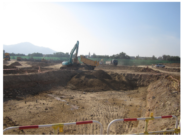
Photo 02 – The treated soil was started to backfill to the proposed location.
