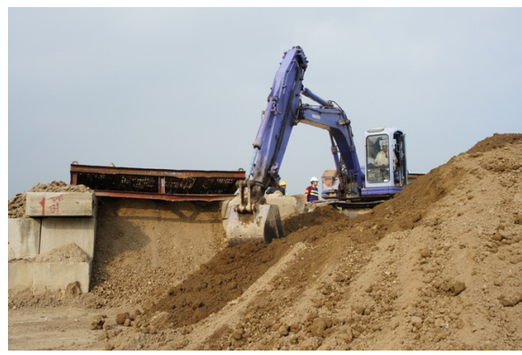
Photo 02 – Excavator was used to loosen the contaminated soil.
