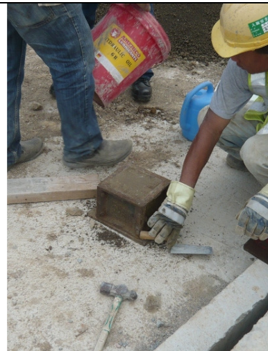
Photo 10 – Preparation of concrete cube.
