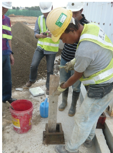
Photo 09 – Preparation of concrete cube.
