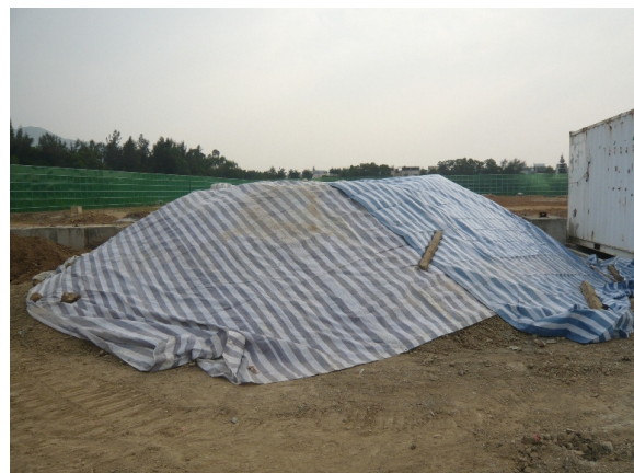
Photo 12 – The treated soil was covered with tarpaulin sheet and placed at a paved area for temporary storage.
