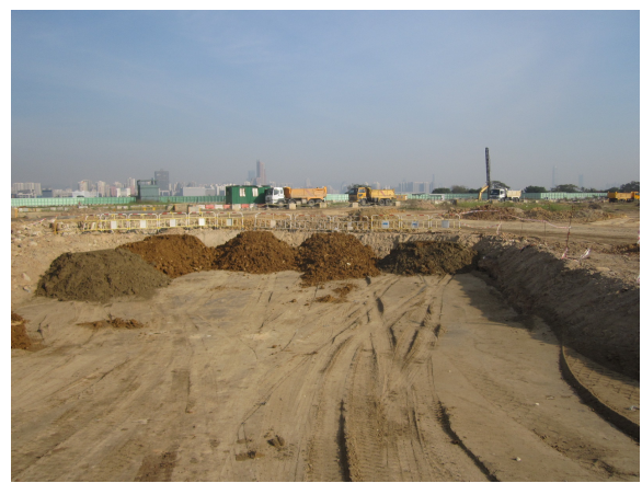
Photo 04 – The treated soil was covered by ordinary soil.
