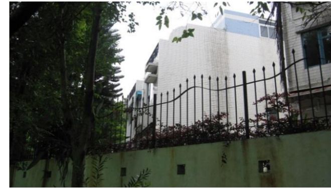
NSR 3 House No. 61, Narcissus Path, Palm Springs
