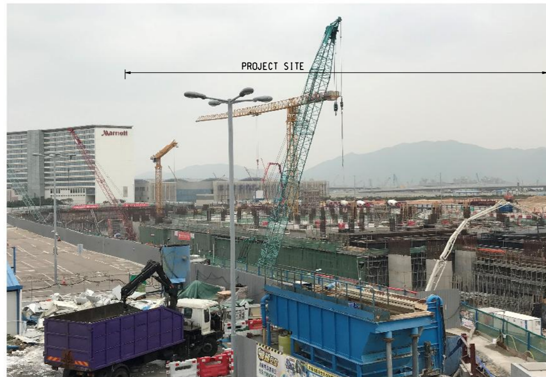
EXISTING VIEW OF O3 AND RE3 FROM NORTH COMMERCIAL DISTRICT
