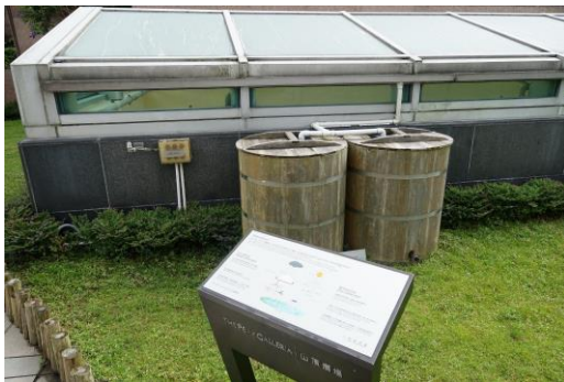
Photo 3: Rainwater harvest system (Photo credit: Green Power)
