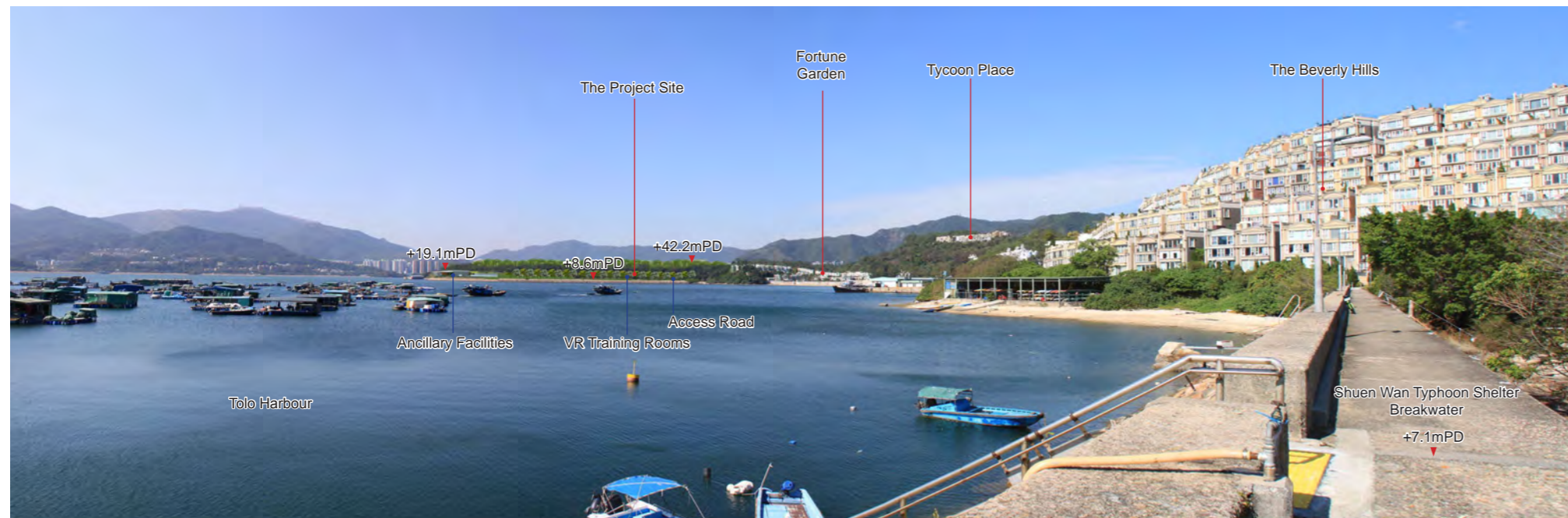
Year 10 of Operational Phase with landscape and visual mitigation measures fully established This image illustrates the screening effect, the Project integrated with waterfront context upon full establishment of planting works.
