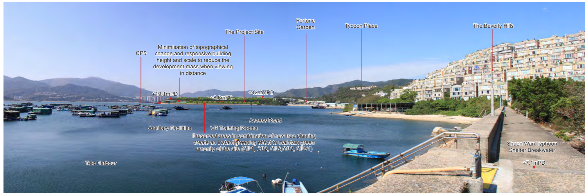
Day 1 of Operational Phase with landscape and visual mitigation measures
