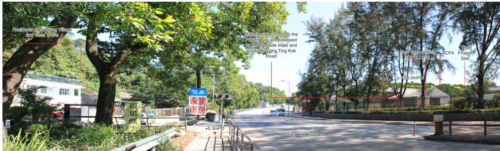
Day 1 of Operational Phase with landscape and visual mitigation measures
