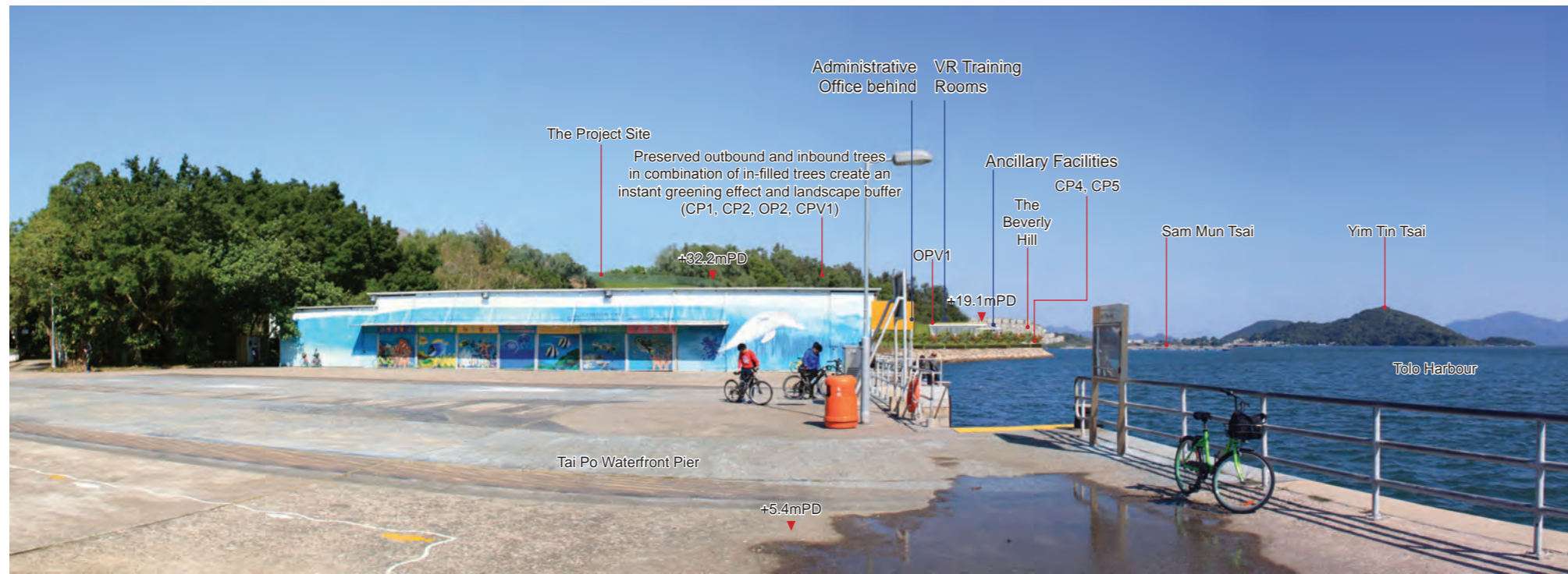
Day 1 of Operational Phase with landscape and visual mitigation measures
