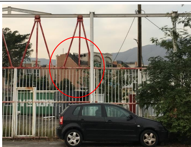
NSR N04. Low-rise residential building, Block 7, Season Monarch
