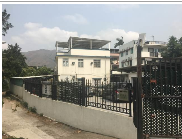
NSR N32. Village house, 1 Wang Toi Shan Lo Uk Tsuen
