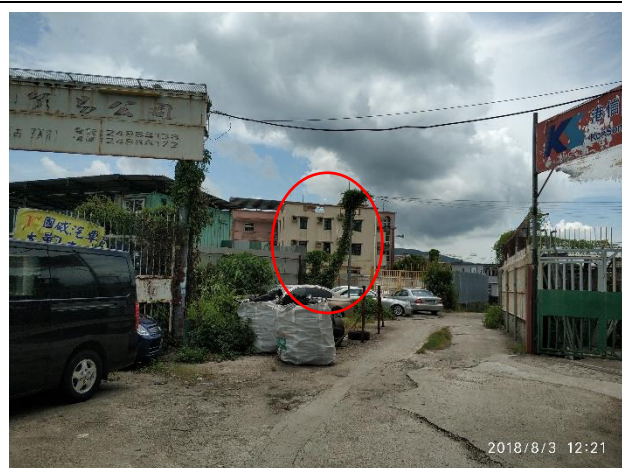
NSR N27. Village house, 94B Wang Toi Shan San Tsuen
