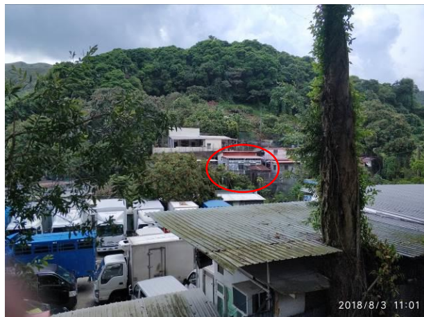
NSR N50. Village house of Wong Chuk Yuen
