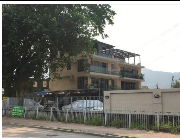
NSR N22. Village house, 28C Wang Toi Shan San Tsuen
