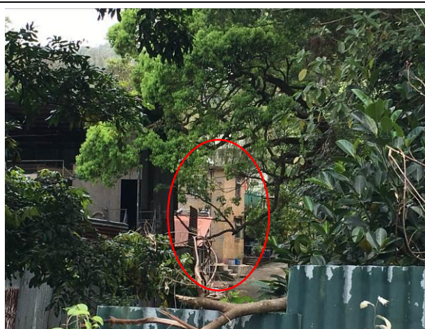
NSR N52. Village house of Wong Chuk Yuen
