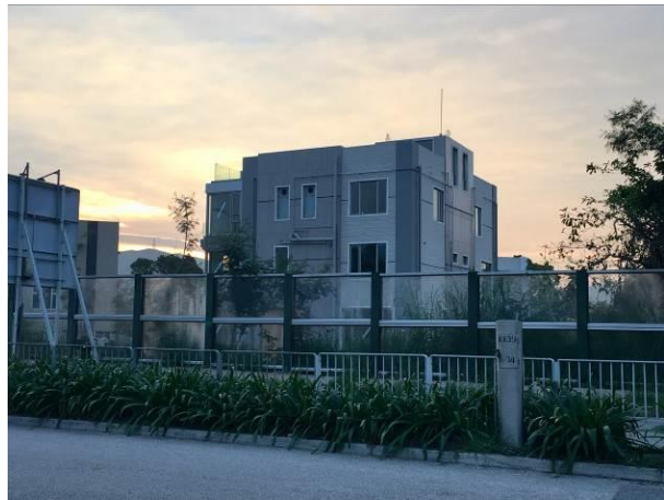
NSR P02. Village house of Wing Lung Wai (under construction)
