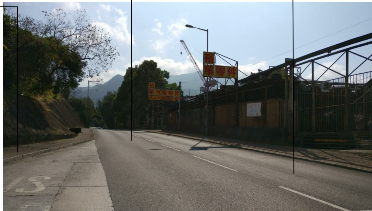
Vantage Point E (Existing Condition)
