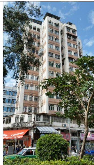
NSR16 – On Ning Building
