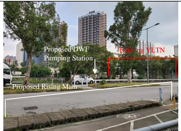
Plate 6: R6 - Tung Tau Wai San Tsuen View to existing YLTN and proposed DWF pumping station is mainly screened by trees planted along YLTN but there is no obstruction for view to proposed rising main.
