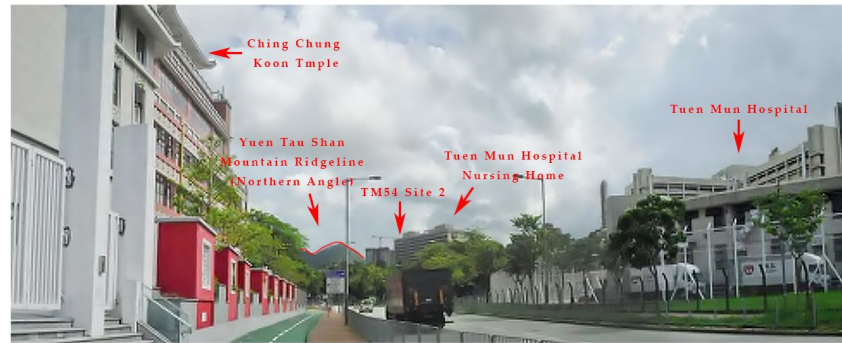
VSR8 Existing View from Tsing Chung Koon Road
