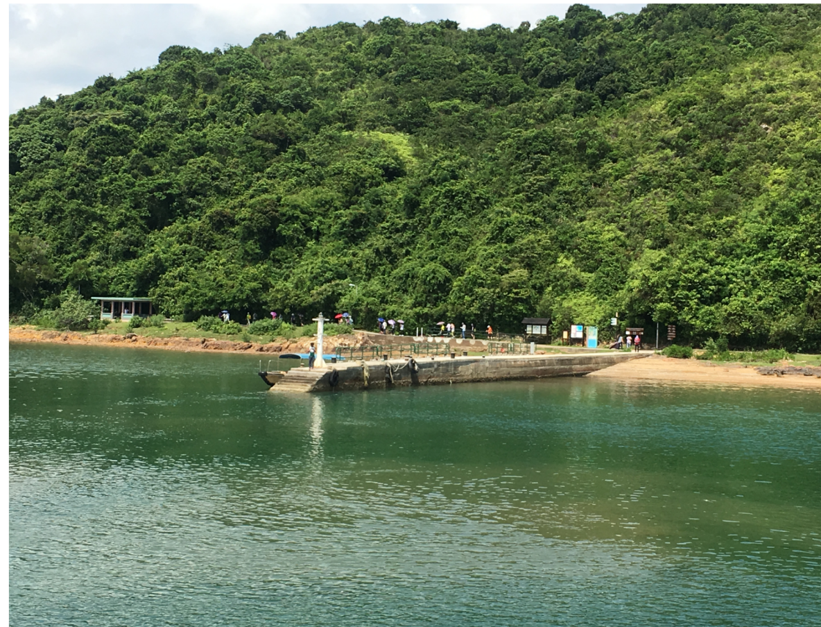
LR8 - LAI CHI WO PIER
