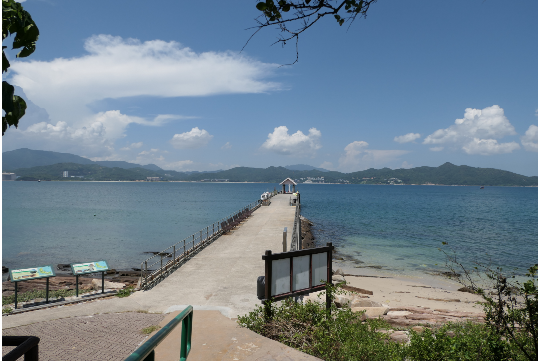
VPA1 - VISUAL CONTEXT OF VSR1 (VISITORS AT THE PAVILION AT WONG YE KOK) TOWARDS NORTHEAST DIRECTION
