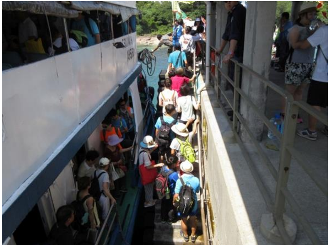
Figure 2.4 Existing Narrow and Steep Landing Steps of Tung Ping Chau Public Pier
