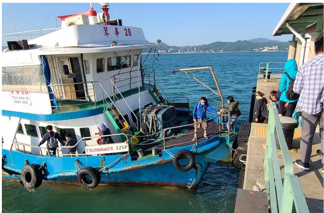
Figure 2.5 Undesirable berthing at the Boat Bow of Existing Tung Ping Chau Public Pier
