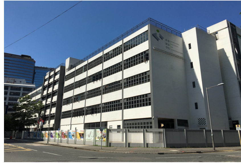
E01 - Construction Industry Council Kowloon Bay Training Centre (CIC Kowloon Bay)
