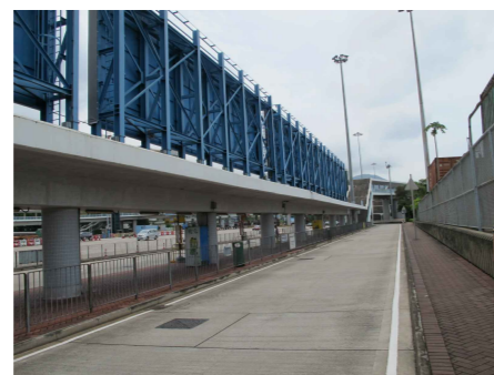
PHOTO 465: ACCESS ROADS AND PEDESTRIAN WALKWAY (PROPOSED FLYOVER ALIGNMENT) (DATE TAKEN: 11 JULY 2019)
