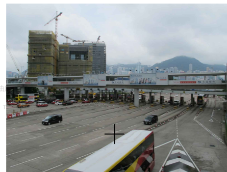
PHOTO 292: TOLL PLAZA OF THE WESTERN HARBOUR CROSSING (DATE TAKEN: 11 JULY 2019)
