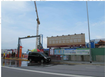
PHOTO 512: HONG KONG PALACE MUSEUM UNDER CONSTRUCTION (DATE TAKEN: 11 JULY 2019)
