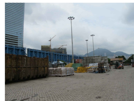
PHOTO 444: STORAGE OF SHIPPING CONTAINERS / CONSTRUCTION MATERIALS AND OPEN AREA (DATE TAKEN: 11 JULY 2019)
