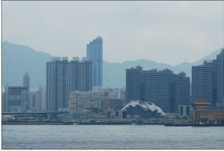
LCA-7 WEST KOWLOON STATION ONGOING MAJOR DEVELOPMENT LCA
