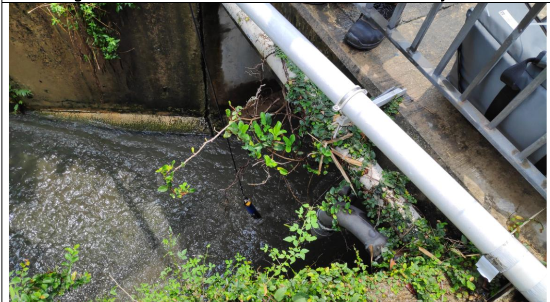
Monitoring Location at HC2 - Downstream of HC Nullah
