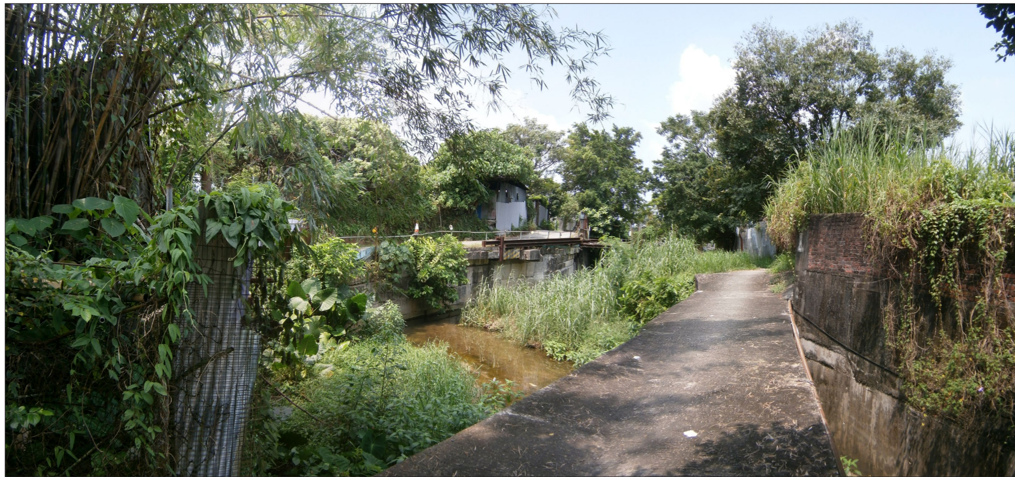
Vantage Point 1: Pedestrians using channel footbridge (VSR 2) (Existing Situation)
