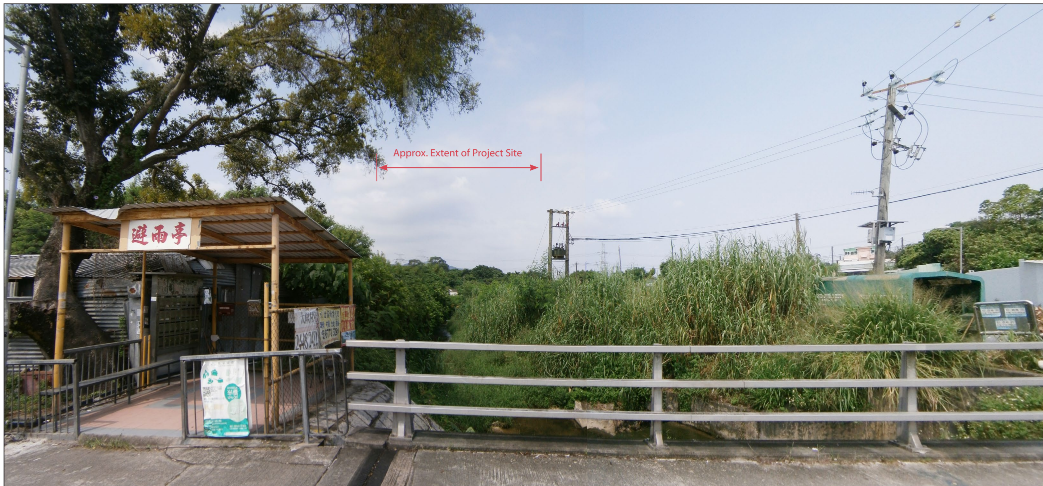
SSNV-VSR8: Vehicle travellers and pedestrians on channel bridge crossing
