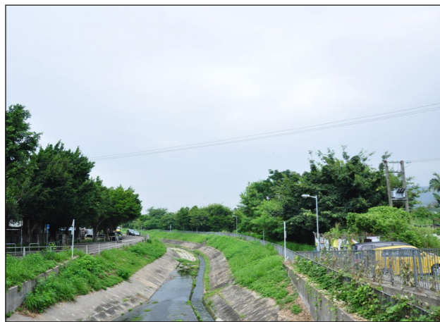
LFT-LCA01: CHANNELISED RIVER CORRIDOR LANDSCAPE
