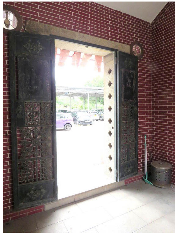
Internal view of GB-04, showing round holes above lintel, tanglung holes for wooden sliding fence on granite door frame, and metal shutters.
