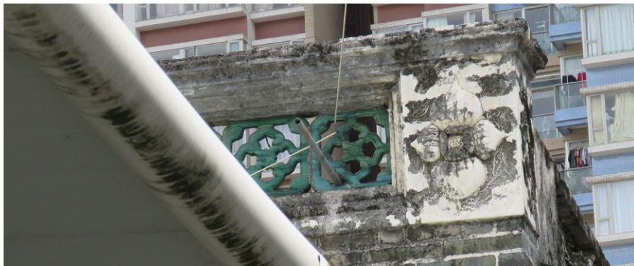
Ceramic grilles and plaster moulding on north elevation.
