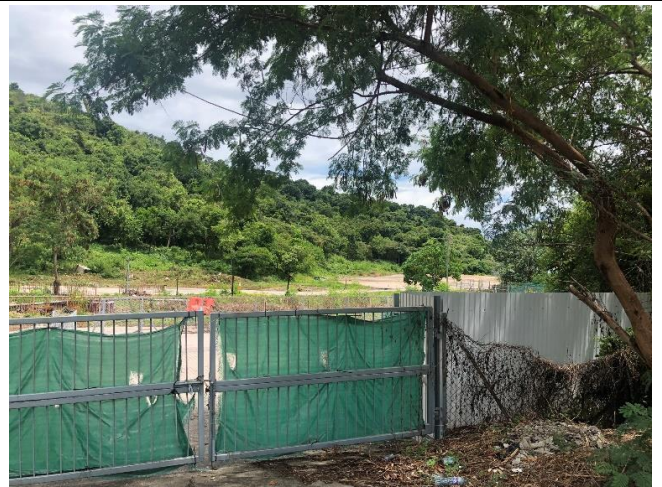
Plate 4 – N3: Existing Condition of the Proposed School with Recreational Area under the Approved Planning Application No. A/MOS/125 (viewed from footpath from Nin Ming Road to seafront)
