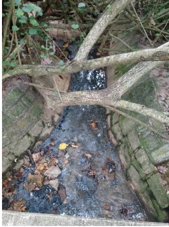
Modified Watercourse W3
