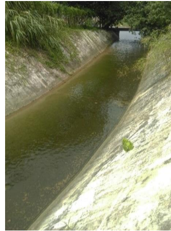
Modified Watercourse W2
