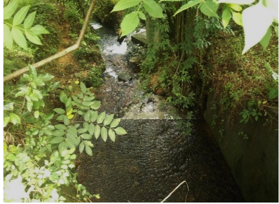
Watercourse W4 (modified upper section)
