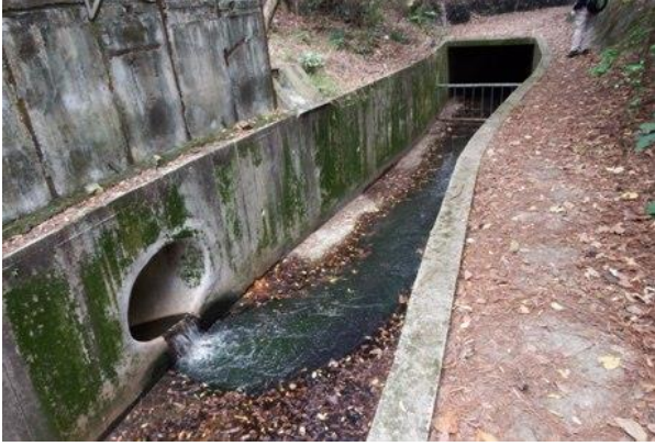
Modified Watercourse W7
