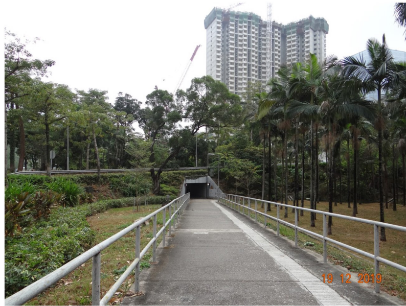
LR3.9 PO KONG INTERCHANGE REST GARDEN
