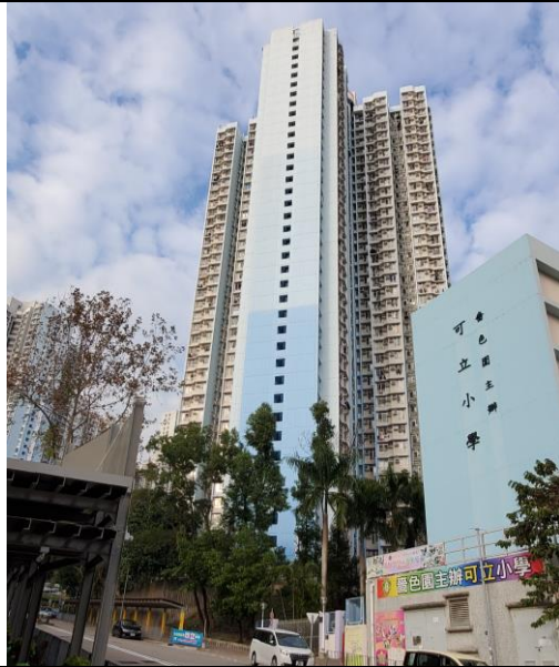
NSR 23 - Lok Shing House, Tsz Lok Estate
