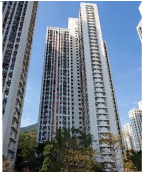
NSR 4 – Chun Wai House, Tin Ma Court
