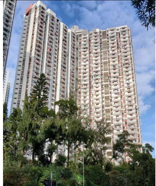
NSR 12 – Mui Yuen House, Chuk Yuen North Estate
