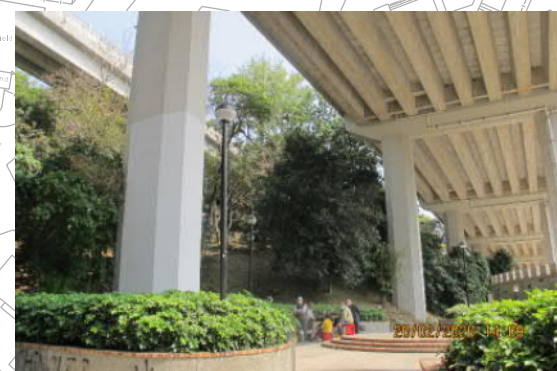
PHOTO 2724: POK NGAR VILLA AND VEGETATION (DATE TAKEN: 20 FEBRUARY 2020)
