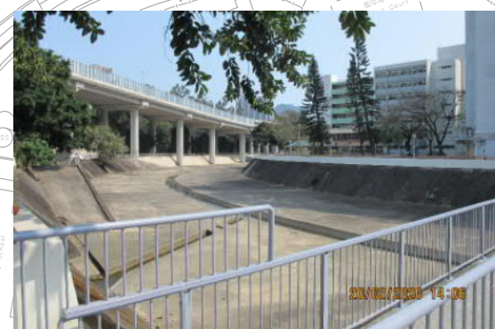
PHOTO 2716: FOOTBRIDGE AND SHING MUN RIVER CHANNEL (DATE TAKEN: 20 FEBRUARY 2020)
