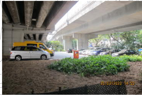
PHOTO 2777: PUBLIC CAR PARK (DATE TAKEN: 20 FEBRUARY 2020)
