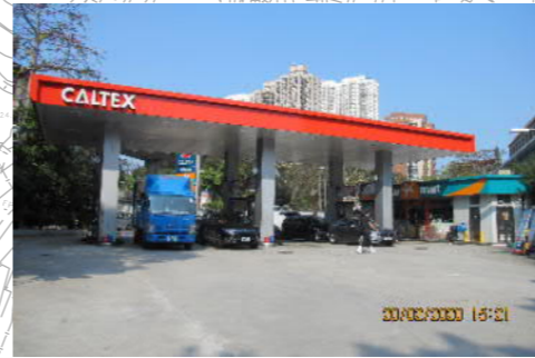
PHOTO 2806: PETROL FILLING STATION (DATE TAKEN: 20 FEBRUARY 2020)
