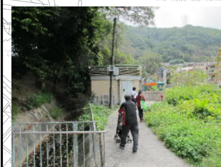
PHOTO 8338: PUBLIC TOILET /NULLAH (DATE TAKEN: 25 FEBRUARY 2020)
