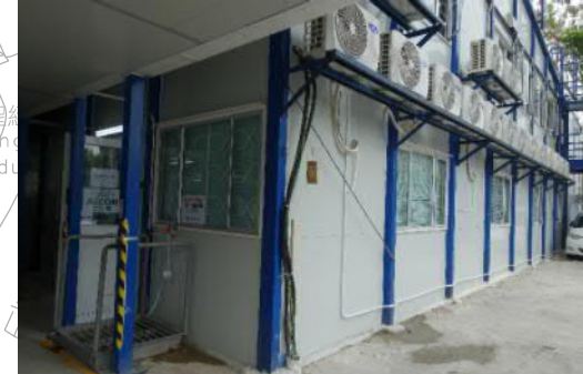
PHOTO 1896: CEDD'S SITE OFFICE (DATE TAKEN: 25 FEBRUARY 2020)
