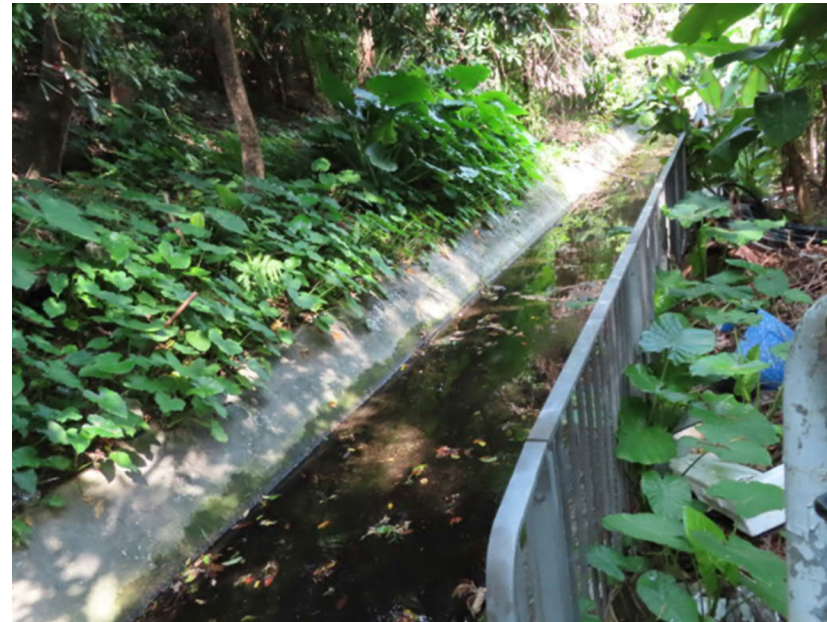
LR-2.3 MODIFIED WATERCOURSE IN SHA TIN TAU
