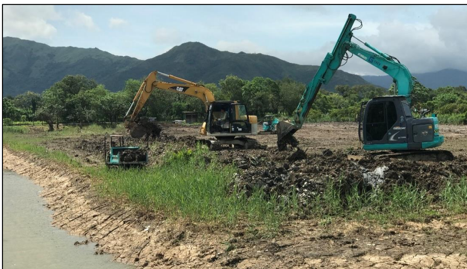
Photograph 2-7 Excavators Working on Drained-down Gei Wai
