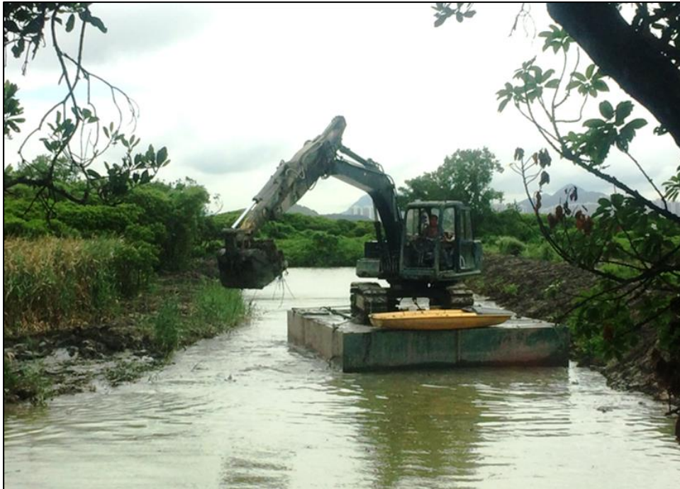
Photograph 2-3 Desilting Channel (from Land)
