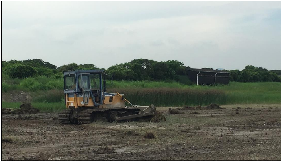
Photograph 2-6 Transferring Material during Drain-down of Gei Wai
