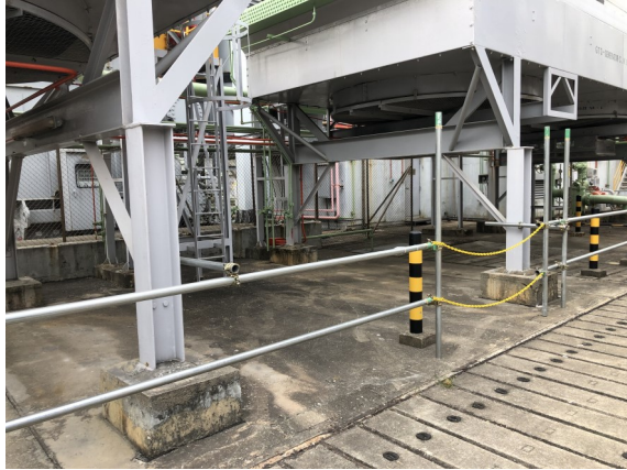
Photo 7: Footings of Generator Coolers
