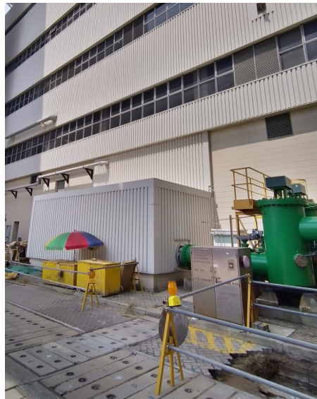
Photo 18: Circulating Water Pipe Room at the immediate east of GT57 Auxiliary Building
