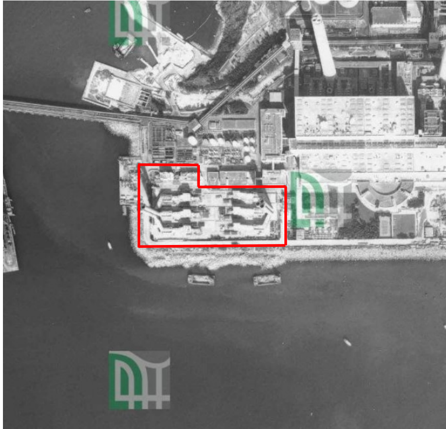
Year 1995: Construction of 6 gas turbines was completed.
