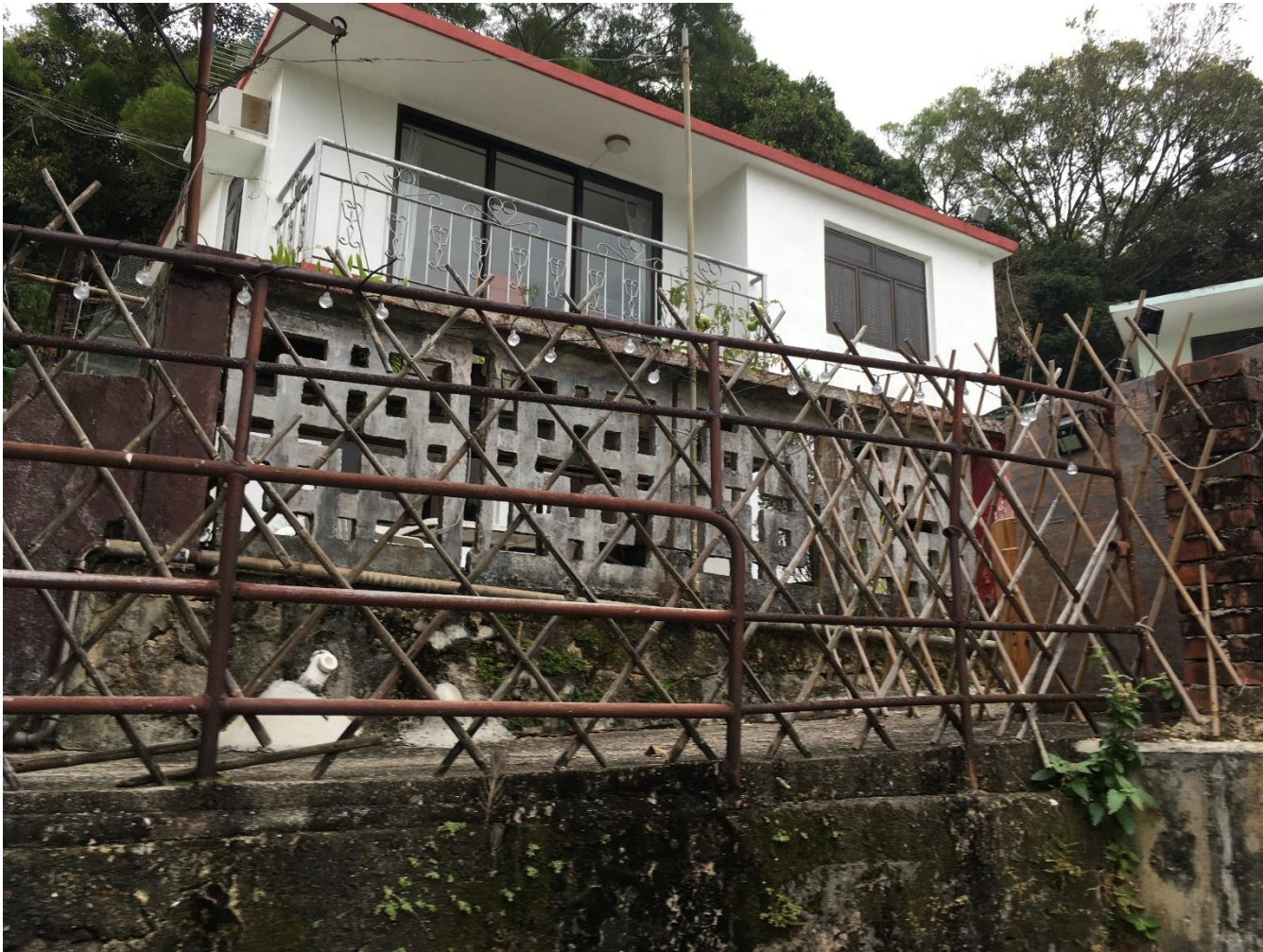
NSR N1 (Village House at Tai Shan Central)
