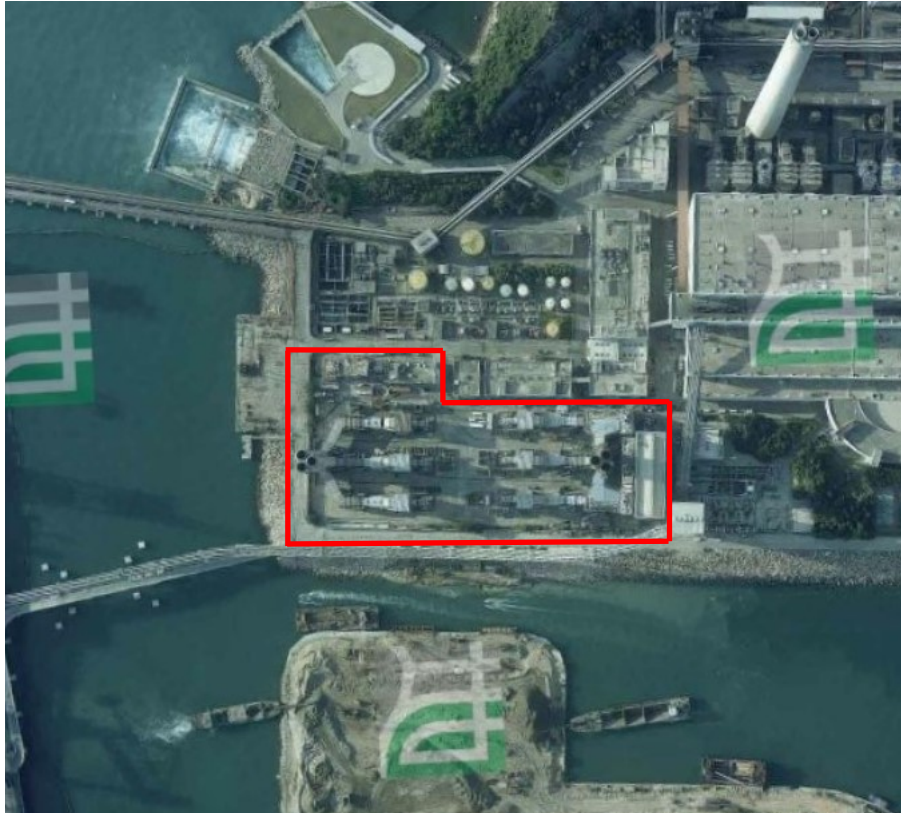
Year 2002: Construction of the GT57 Auxiliary Building was completed.
