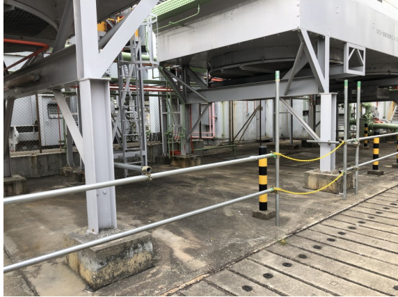
Photo 7: Footings of Generator Coolers
