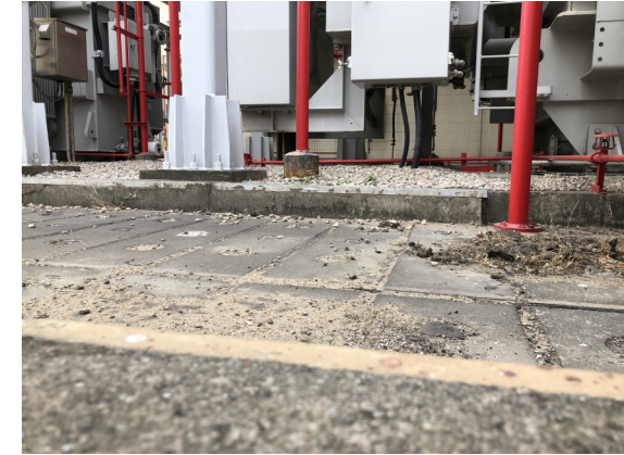
Photo 9: GT's transformer concrete paved ground
