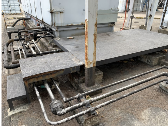
Photo 11: Diesel supply pipes
