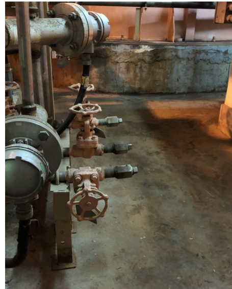
Photo 17: Main oil tank paved surface in good condition
