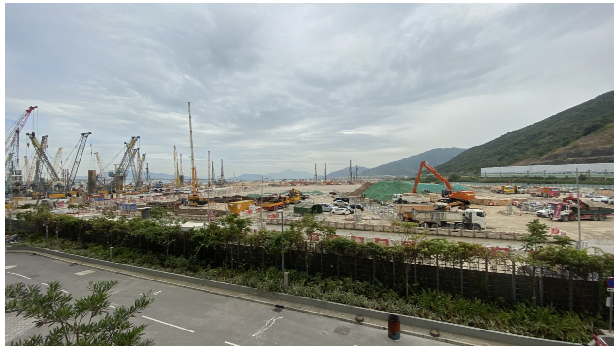
LR16 ONGOING RECLAMATION AREA
