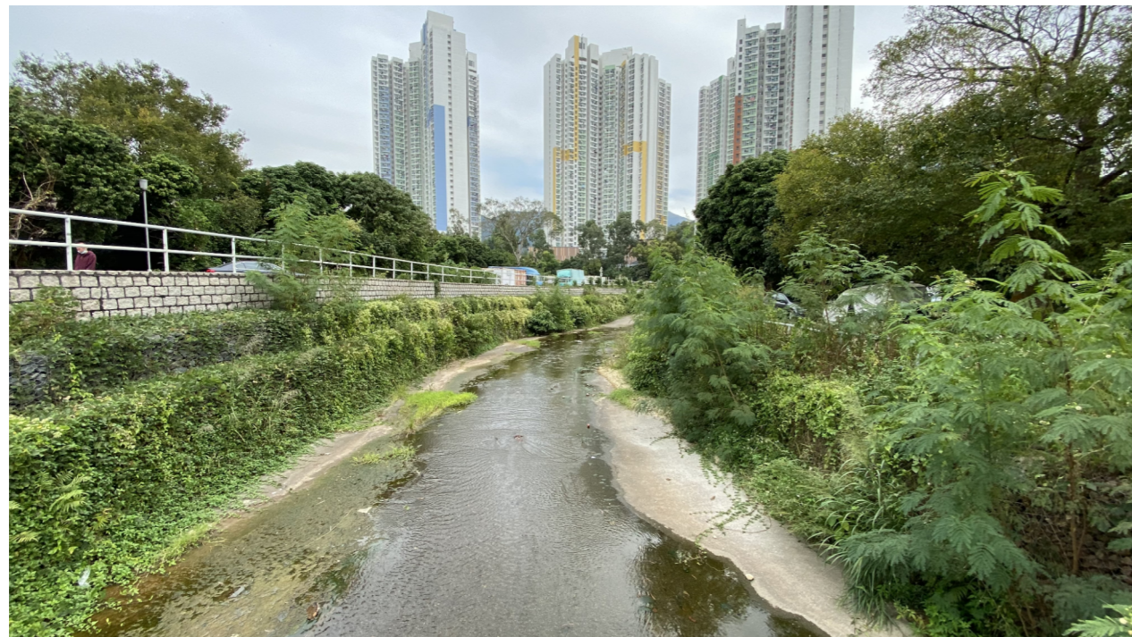
LR10b CHANNELIZED WATERCOURSE
