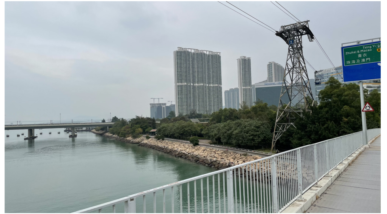
LR12 ARTIFICIAL SEAWALL
