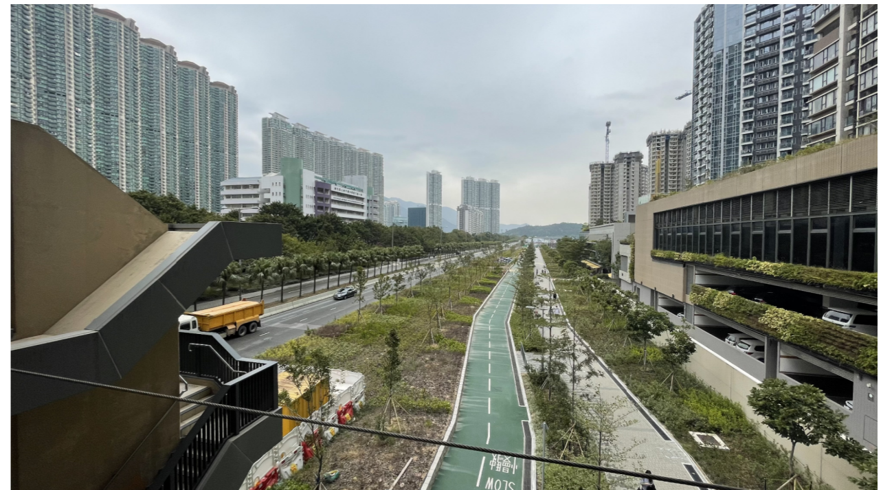
LR13b ROAD AND INFRASTRUCTURE
