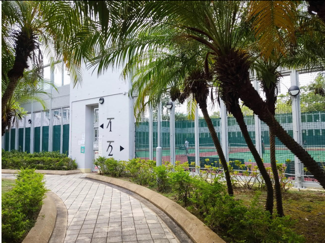
View Point F – Wu Shan Tennis Court
